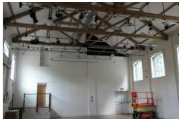
Further framework for lighting installed above stage.
